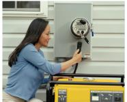
tomatically disconnects from the utility grid, preventing electricity from traveling back out onto the line.
